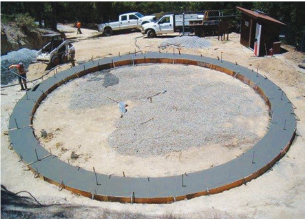
The Idyllwild Water District is constructing a new 200,000-gallon water storage tank for its Golden Rod well. The new tank ring foundation pad (shown) required 40 yards of poured concrete. Steel construction will begin next Wednesday to allow the foundation to cure.
