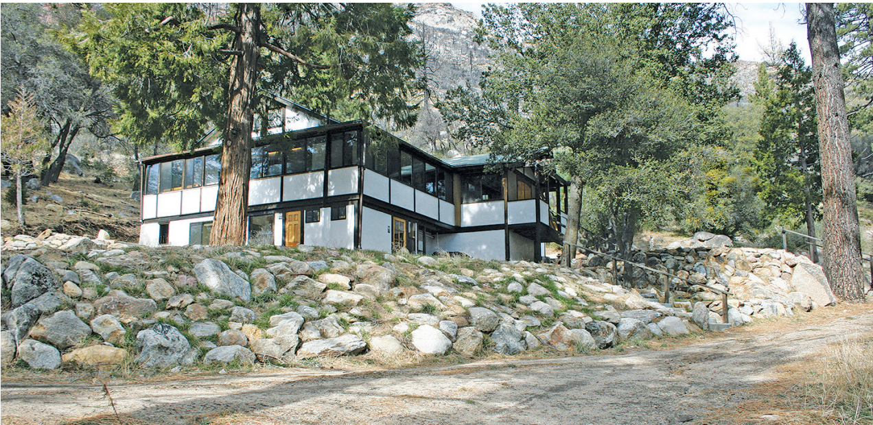
Tons of mud and debris were used to elevate the “yard” of one of the center buildings about 4 feet, fortified with rocks carried by the floods that followed the Mountain Fire of 2013. With the elevated “yard,” the building is better prepared to withstand future major flooding. “We prioritized protecting the center’s buildings at the expense of the roads,” said Abbot Tenshin Fletcher, Roshi . PHOTOS BY MARSHALL SMITH
