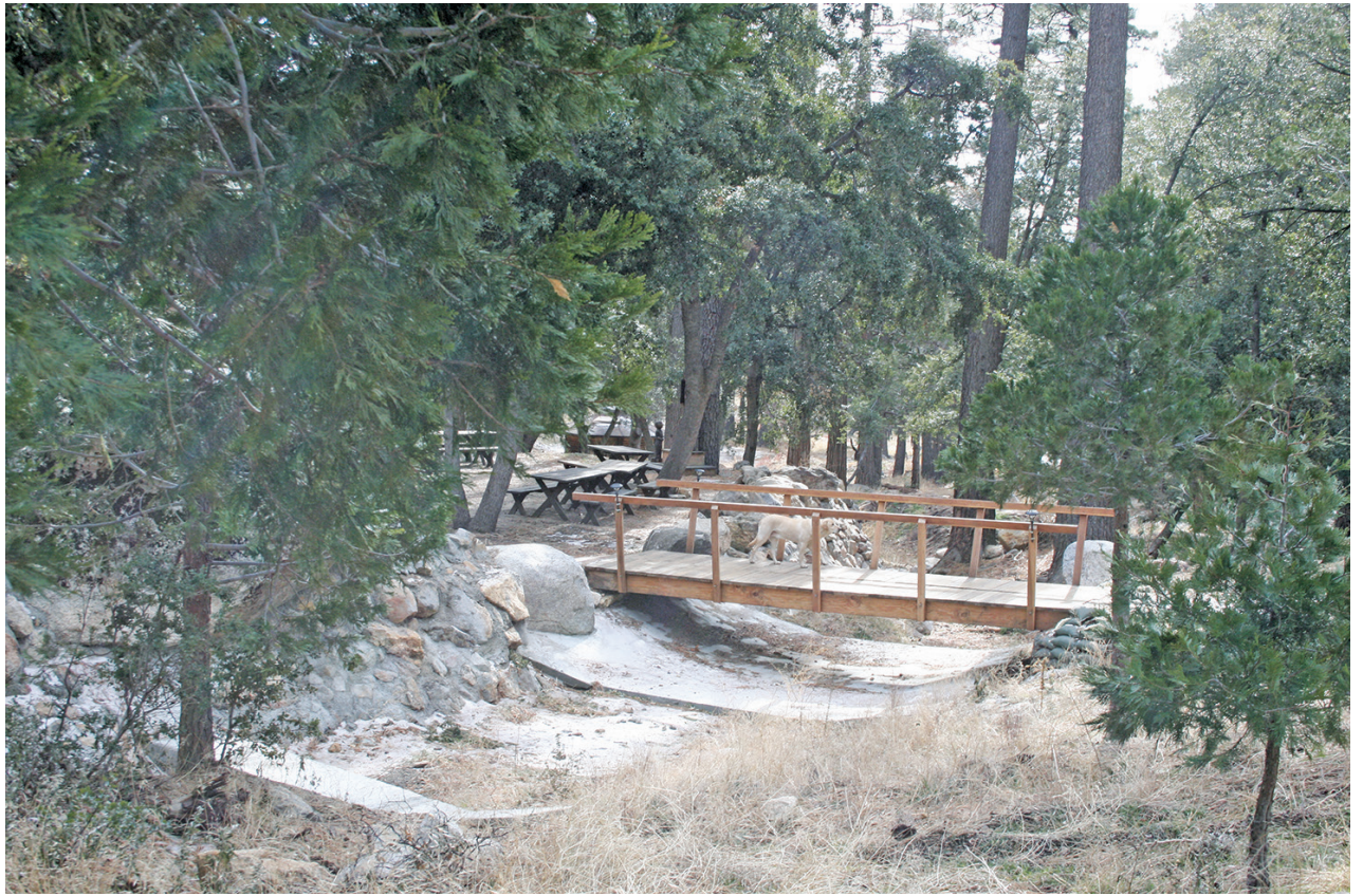
A newly constructed water course fortified with concrete and a walk bridge that can flip open into two sections to avoid water damage. PHOTO BY MARSHALL SMITH
