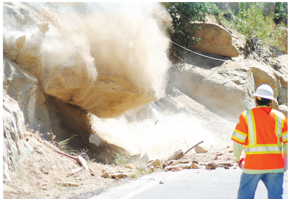
One of two boulders above Highway 243 at Deadman's Curve in Pine Cove is pulled off the steep slope on Wednesday morning. A Caltrans team is removing these so they do not fall unexpectedly on the highway, as one did last January. The crew used air bags to push the second boulder onto the highway. PHOTO BY JP CRUMRINE
