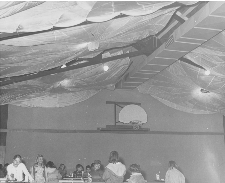
A new use for parachutes in January 1962 was an effort to improve acoustics in the multipurpose room at Idyllwild School. Eight chutes were installed at a cost of about $8. Results indicated some improvement.
