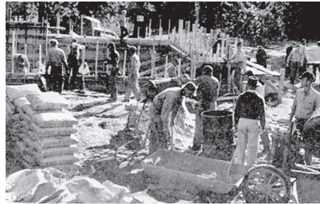
Volunteers pouring the foundation for Town Hall in 1946.
