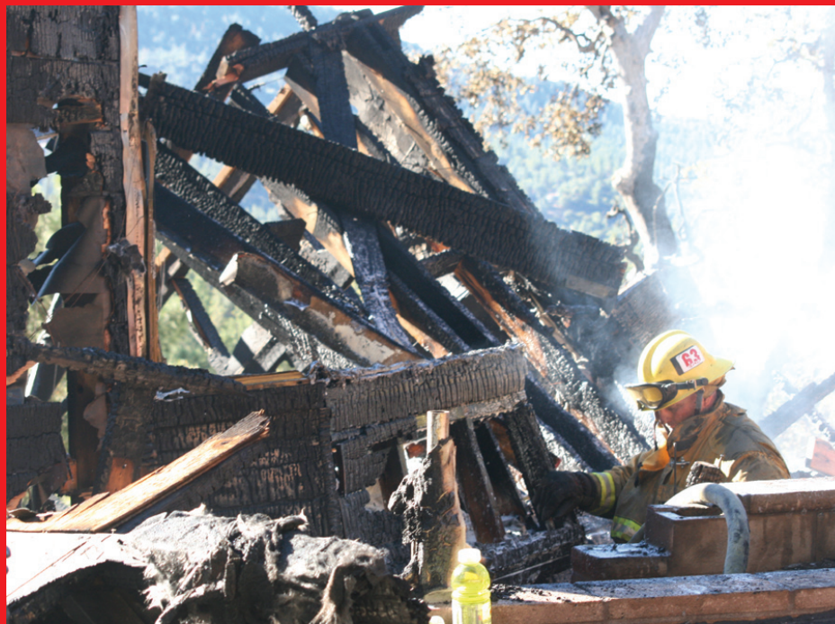
A firefighter emerges from the smoking ruins of a once beautiful home on Foster Lake Road. PHOTO BY MARSHALL SMITH
