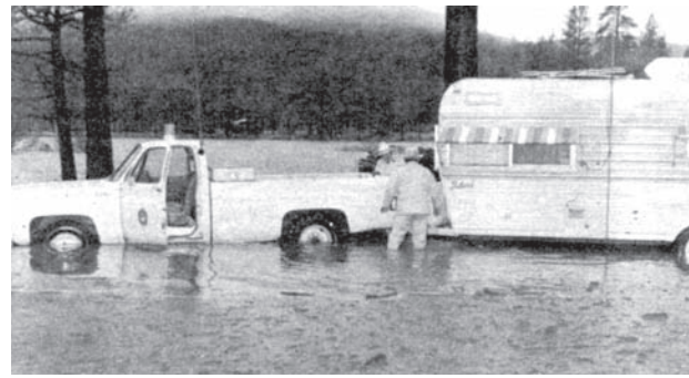
In February 1980, a 5-day storm dumped more than 9 inches of rain on the Hill. Lake Hemet reached its highest level since the dam was built in 1889. Here, the Lake Hemet crew is rescuing one of 16 trailers from the flooded campground.
