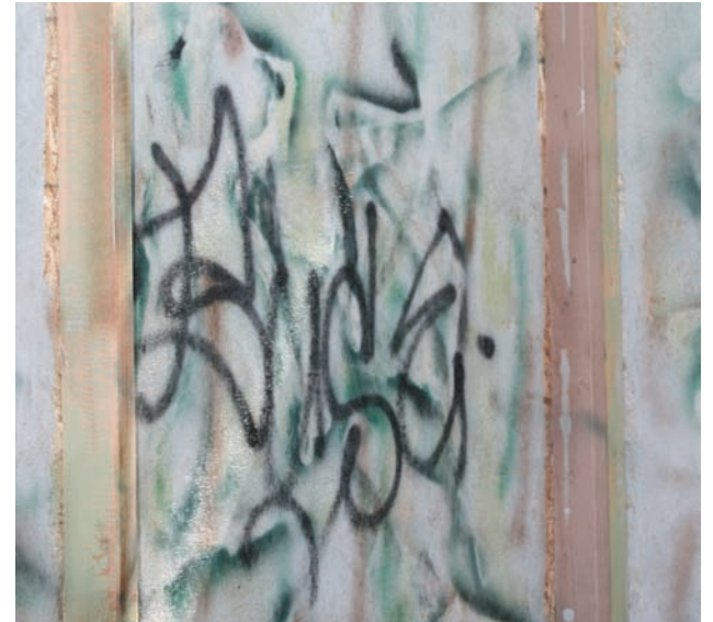
Vandals broke into the Idyllwild Haunted Ghost Town on Thursday, Sept. 23 and sprayed graffiti on several wall panels and a hanging drape. PHOTO BY MARSHALL SMITH
