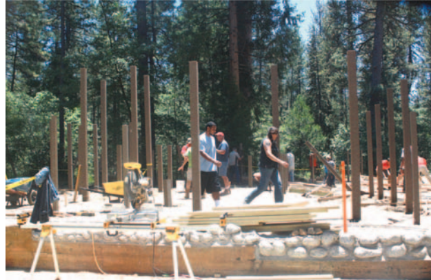
The posts start going up for the maze on the first day of the playground build at the Community Center site. At right, the structure steeples are constructed.
