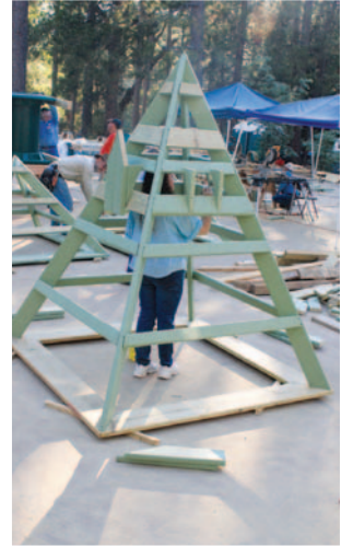
The posts start going up for the maze on the first day of the playground build at the Community Center site. At right, the structure steeples are constructed.
