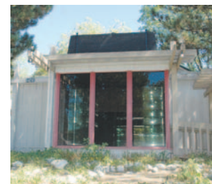
A vacant storefront in a prominent location.
