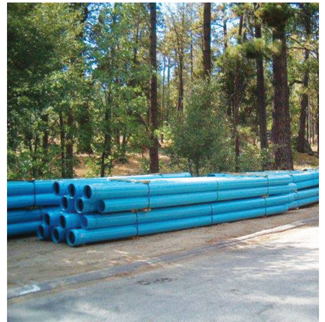
Inland Backhoe is installing 2,500 feet of 8-inch pipe for Idyllwild Water District's new storage tank in the Toll Gate Zone. It will take about two and half weeks to install this pipeline.
