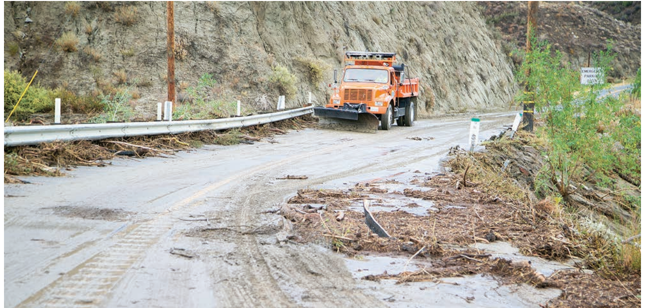
Sunday's wet storm brought mud and debris flooding onto Highway 74 near mile marker 49, completely shutting down the road in both directions for most of the afternoon. Caltrans and the California Highway Patrol were on scene to clean up and direct people to the quickest detour.
