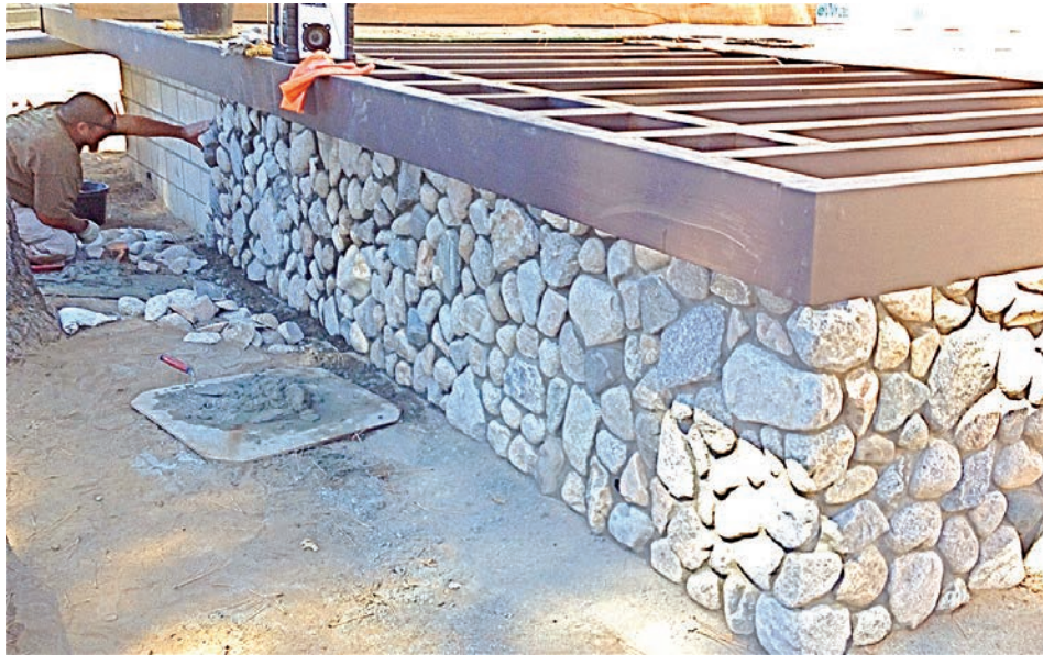
Craig Brock of Roby Gray Construction puts a river-rock facing on the front deck of the new Ferro restaurant on Cedar Street last week.
