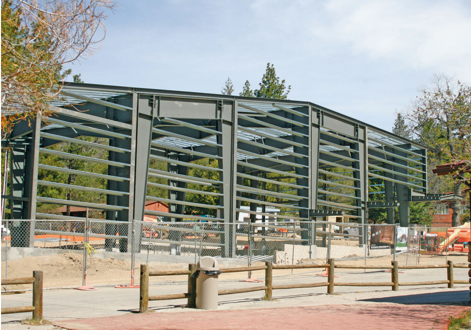
Steel framework is in place for the Lowman Concert Hall on the Idyllwild Arts campus. Completion is anticipated for late August or early September 2015.
