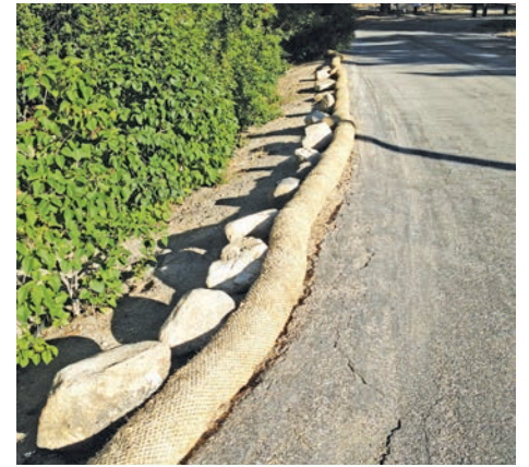
Residents are already preparing for an El Niño winter. Rather than sandbags, this home has a berm protecting it from runoff along the street. PHOTO BY JP CRUMRINE
