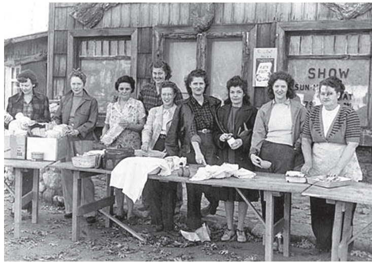
Idyllwild community members built Town Hall from the ground up. PHOTO COURTESY KAT WILSON
