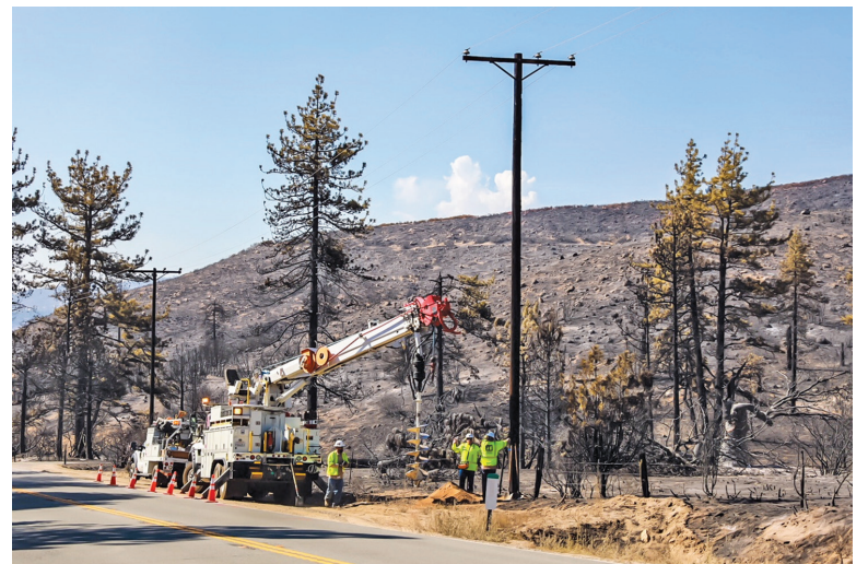
Southern California Edison crews replace power poles damaged or destroyed in the Cranston Fire. PHOTO COURTESY SOUTHERN CALIFORNIA EDISON
