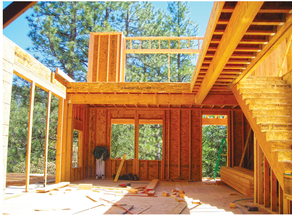
The Grand Idyllwild Lodge under construction. PHOTO COURTESY BRAD RECHTFERTIG
