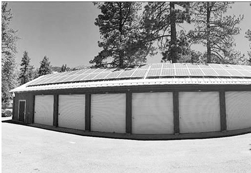
New solar panels on the roof of the U.S. Forest Service's local warehouse help conserve energy and save money.
