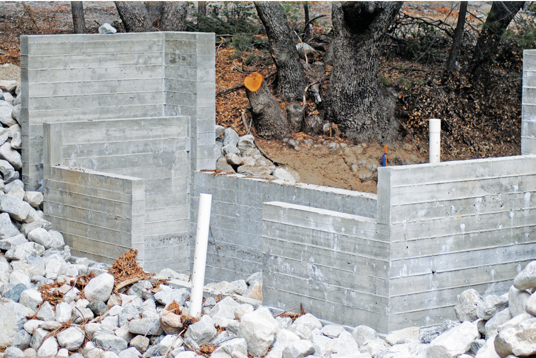
Above, GNW construction of Idyllwild constructed this weir for Idyllwild Water District to measure the flow from Lily Creek into Foster Lake. PHOTO BY JP CRUMRINE Right, to remove the disinfectant by-products in its water, the Idyllwild Water District purchased a granulated activated carbon filter, which is being installed at the District's facilities at Foster Lake. PHOTO BY JP CRUMRINE
