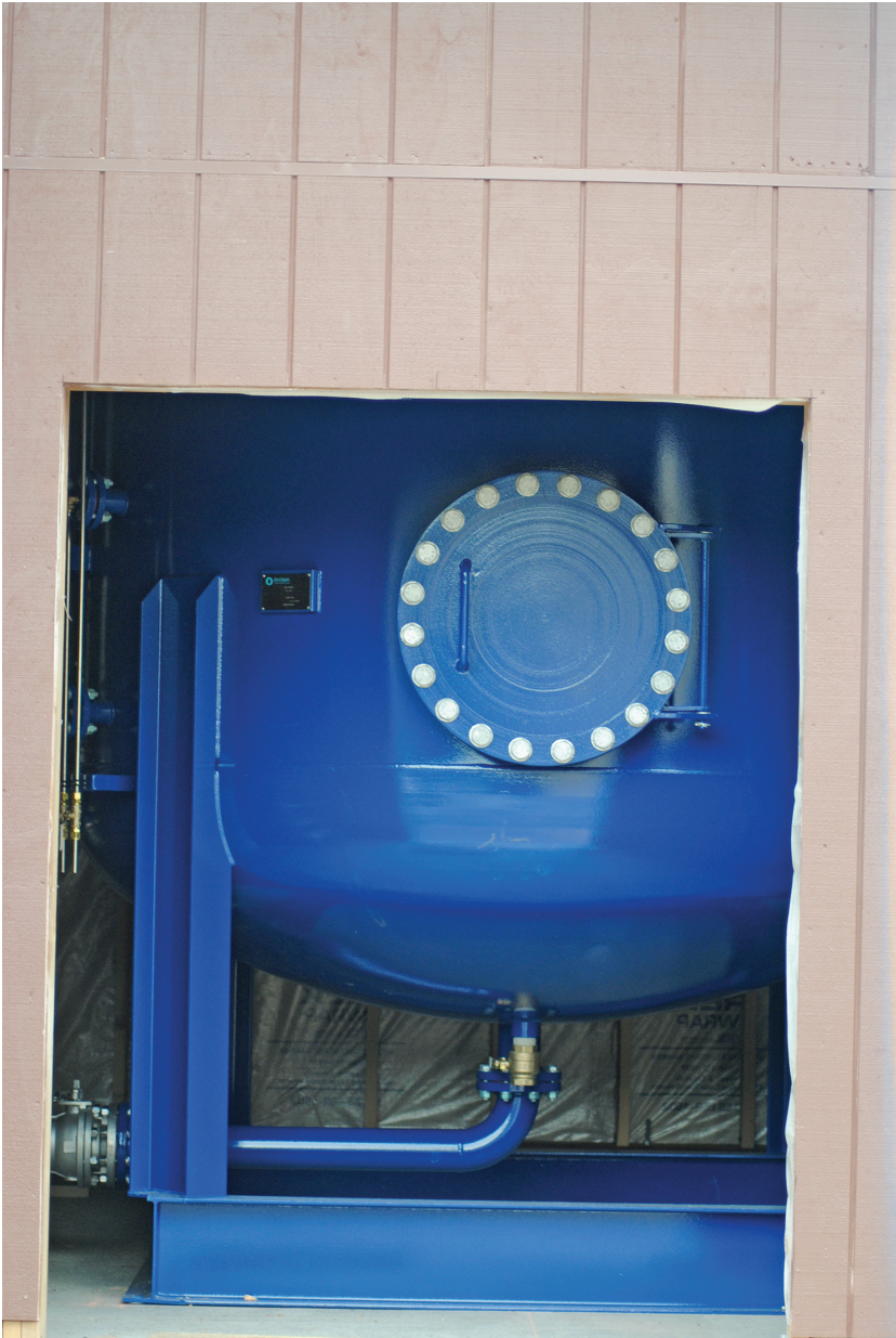
Above, GNW construction of Idyllwild constructed this weir for Idyllwild Water District to measure the flow from Lily Creek into Foster Lake. PHOTO BY JP CRUMRINE Right, to remove the disinfectant by-products in its water, the Idyllwild Water District purchased a granulated activated carbon filter, which is being installed at the District's facilities at Foster Lake. PHOTO BY JP CRUMRINE
