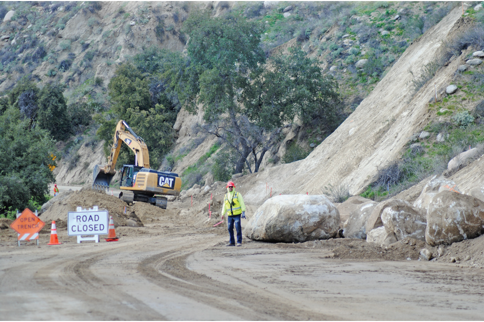
Ames Construction, the Caltrans contractor, is repairing the collapse of Highway 74. As of Thursday, Feb. 28, the re-paving had not started until a satisfactory base has been restored. PHOTO BY JP CRUMRINE
