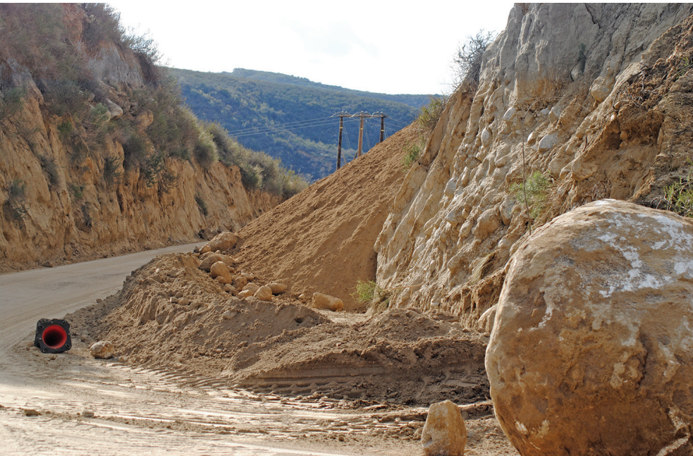
Ames Construction, the Caltrans contractor, is repairing the collapse of Highway 74. As of Thursday, Feb. 28, the re-paving had not started until a satisfactory base has been restored. PHOTO BY JP CRUMRINE
