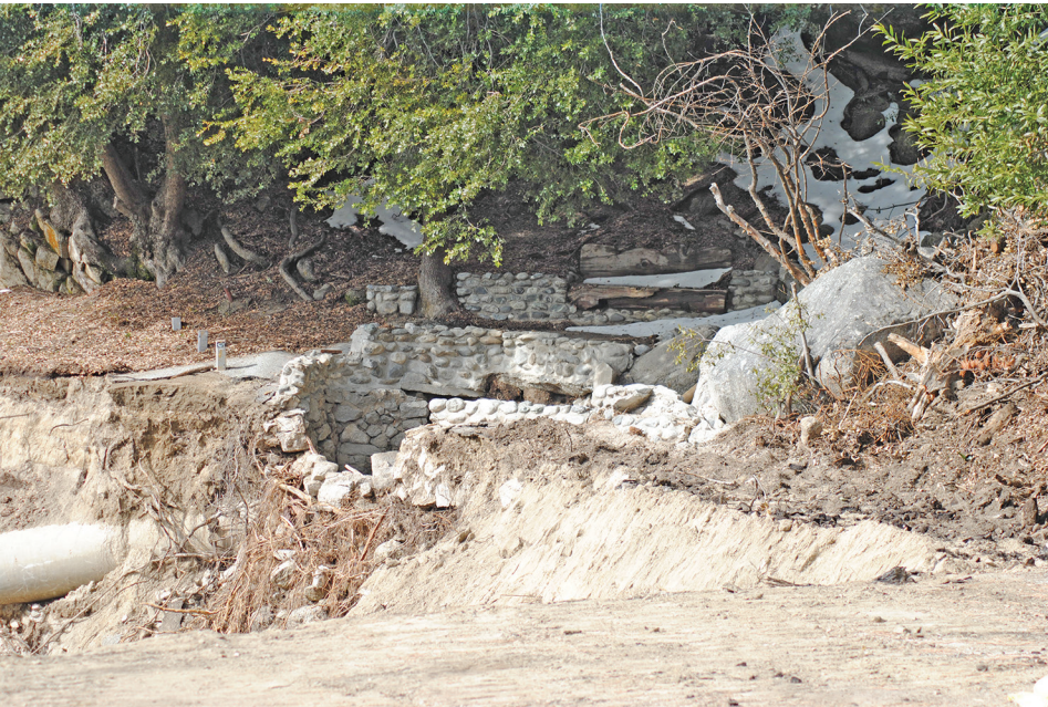
The stone works at the Bay Tree Springs were essentially undamaged although Highway 243 collapsed in front of the spring. The hillside must be restored and compacted before any road surface can be relaid. PHOTO BY JP CRUMRINE
