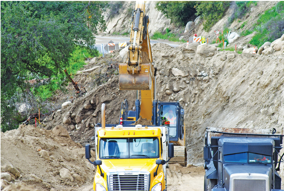
Above: A portion of Highway 74 just west of the Cranston Ranger Station and the Turkey Farm was severed after the Feb. 14, torrential rains. In order to restore the road, the base, which was severely eroded by runoff, has to be rebuilt.
