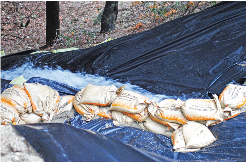
Water flowing from Bay Tree Springs, which had been routed under Highway 243 until it collapsed, had to be diverted so that the road repair could be done.
