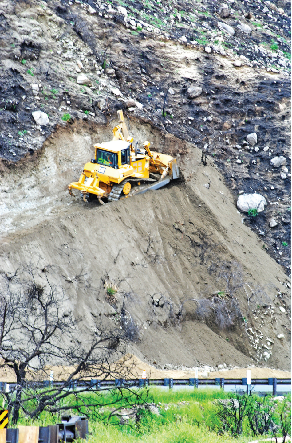
Besides repairing the damaged highway, Caltrans engineers identified several locations where the hillside, or wall of the mountain, posed future danger for rockslides or collapse. Here is work being done to reduce this future risk by scaling the hillside to reduce its steepness.
