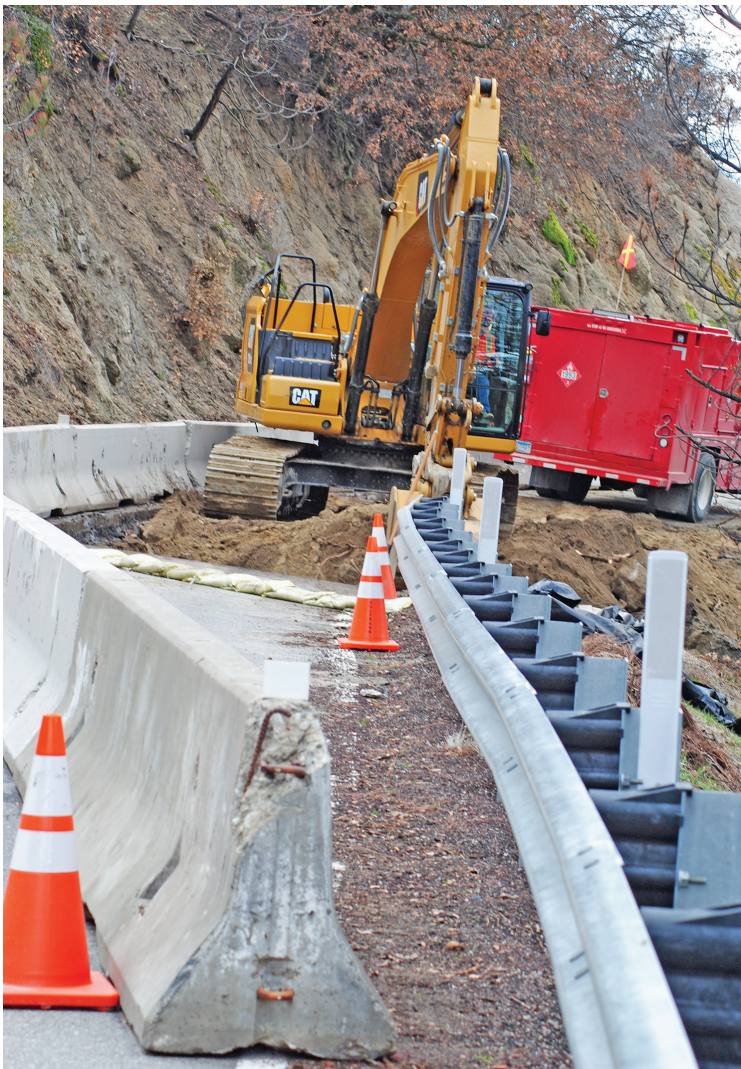
Besides repairing the damaged highway, Caltrans engineers identified several locations where the hillside, or wall of the mountain, posed future danger for rockslides or collapse. Here is work being done to reduce this future risk by scaling the hillside to reduce its steepness.
