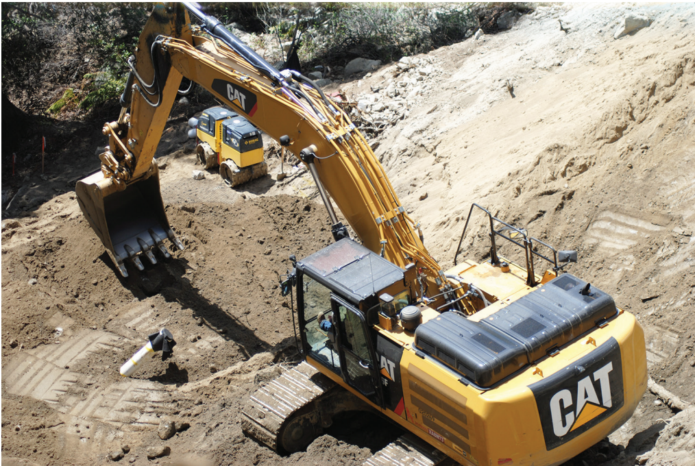
Reconstruction of Highway 243 continues. Here the excavator is used to begin rebuilding the base of the road. The work is about 75 feet below the former road surface.
