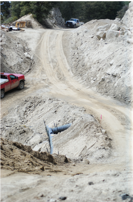
Reconstruction of Highway 243 continues. Here the excavator is used to begin rebuilding the base of the road. The work is about 75 feet below the former road surface.
