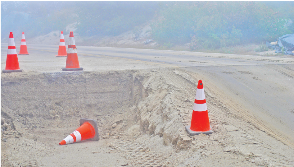
Repair of Highway 243 north of lake Fulmor includes replacing old and small culverts. During heavy rainstorms, these tend to overflow and can damage the road. Replacing the culverts requires excavating about 100 feet of road surface down about 50 feet. This work is being done near milepost 15. PHOTO BY JP CRUMRINE
