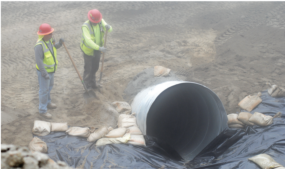
At Bay Tree Spring, Caltrans has to restore and reconstruct the road that washed away. This involves replacing older culverts with newer and larger pipes. This culvert will be about 40 feet below the road surface. PHOTO BY JP CRUMRINE
