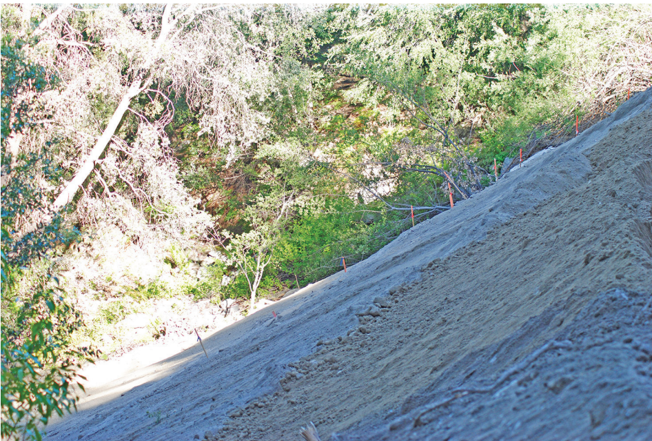
Work on reconstructing Highway 243 at Bay Tree Springs continues to progress. This photo shows how much of the base has been restored since the February washout, which destroyed the road to the trees at the bottom left of the photo. PHOTO BY JP CRUMRINE
