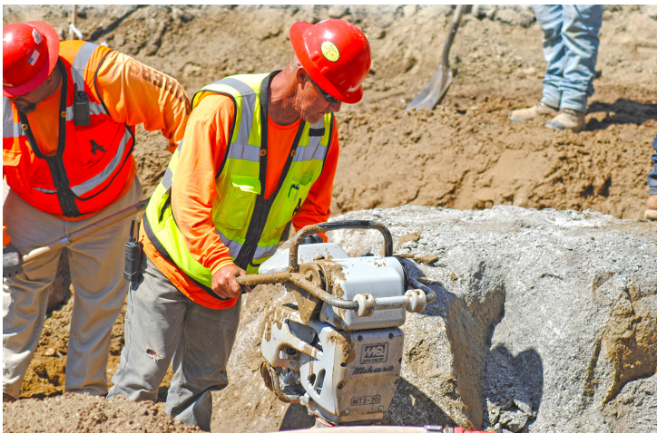
This boulder, which is being broken into smaller pieces, was located just below the road surface of Highway 74. It was discovered when work began on replacing an older culvert, which was eroding the hillside below the road.
