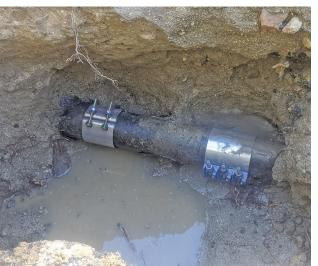
Repair clamps stop a leak.
