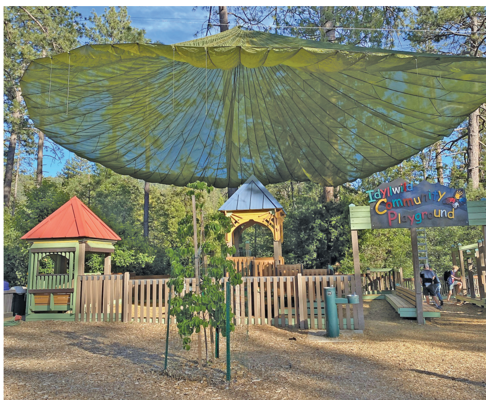
The first of two parachutes was installed by the Idyllwild Community Center Tuesday, June 8 at the Idyllwild Community Playground. The second one is expected to be installed in the near future. PHOTO BY STEPHANIE YOST
