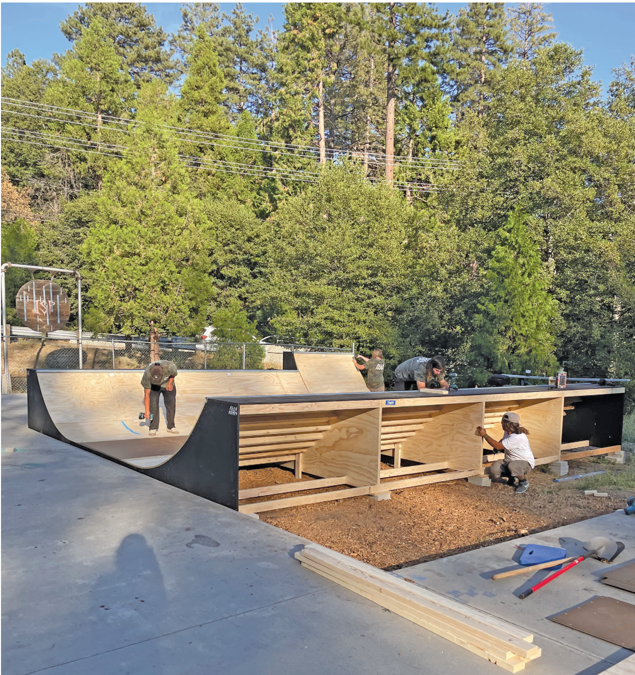
Staff from Keen Ramps install the new half pipe feature at the Idyllwild Skatepark.
