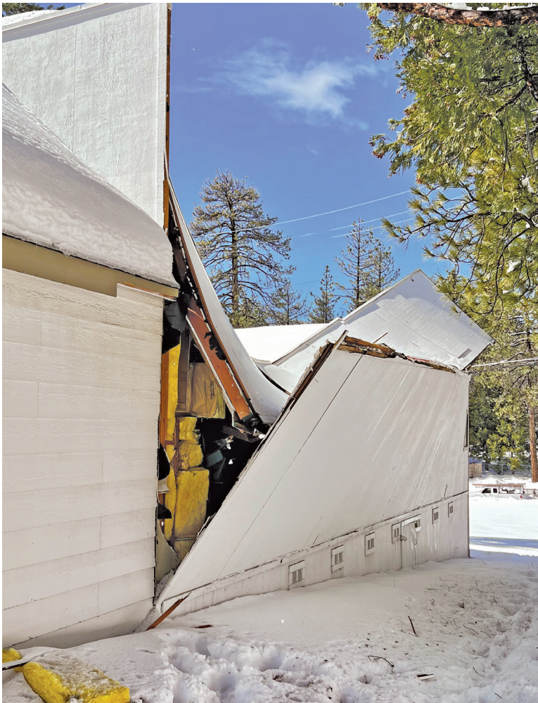
The weight of the snow caved part of the roof at Tarah Jade's during the storm last week.
