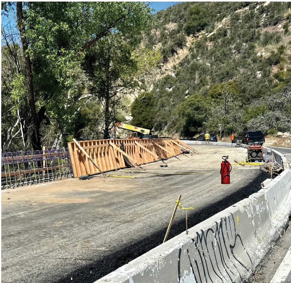
As of Sunday, May 19, Caltrans Constuction on route 74 bridge retrofit at Strawberry Creek will shift gears to the opposite lane.Crews have completed pouring the eastbound abutment and retaining wall for strawberry Creek as of the 19th, additional work includes upgrades with slab overlay, new guard rail systems on the existing bridges, and bringing lane and shoulder width up to current standards. Traffic control will remain the same as it has been just utilizing the opposite lane now as Constuction moves to the other side.Unfortunately, there are quite a few months left to complete overall construction on this project.
