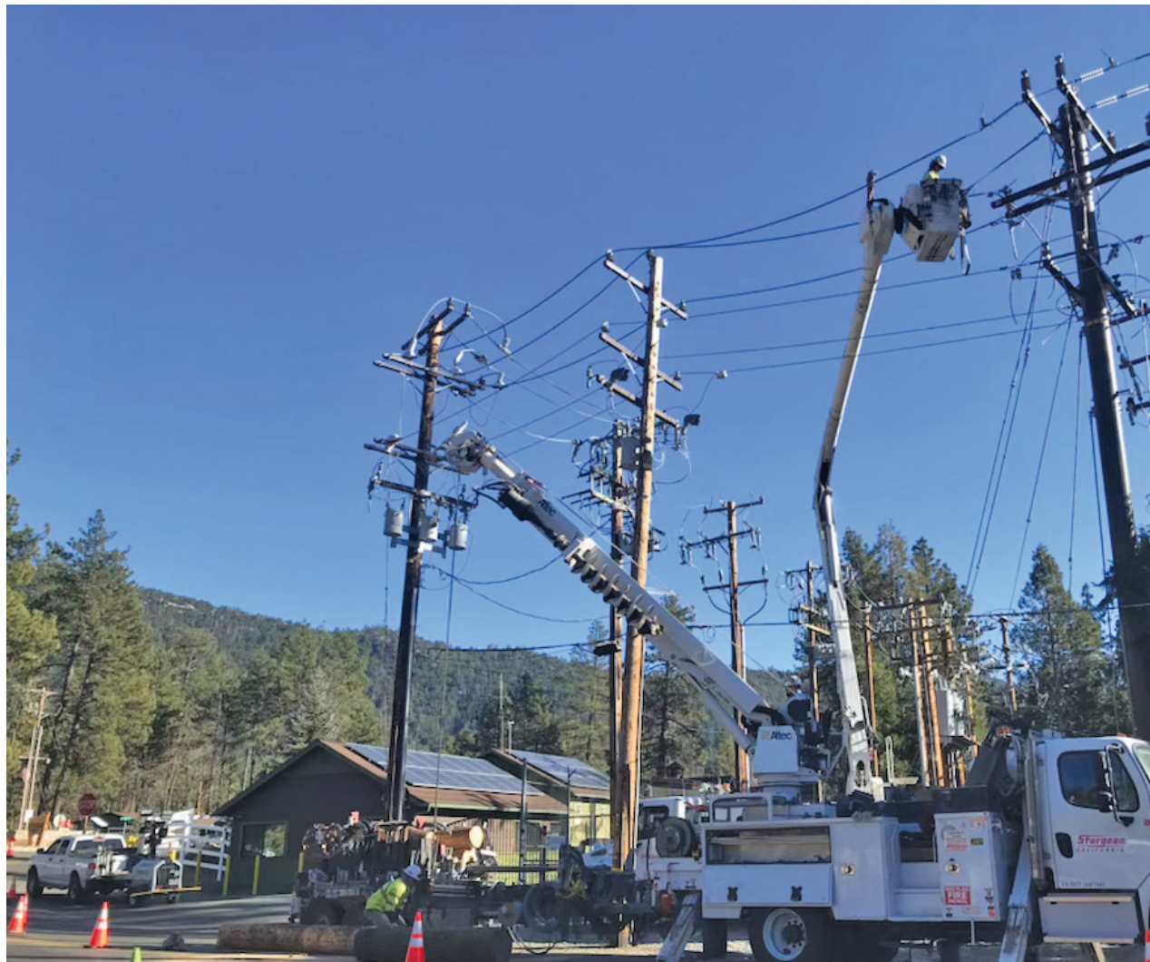
Two line men work above to complete replacement of powerpole.
