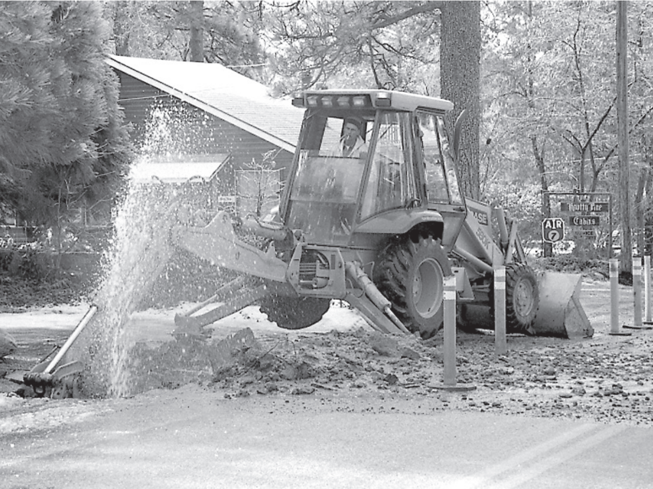
Jim Hamilton, who was an Idyllwild Water District field maintenance worker, digs up a section of Upper Pine Crest to get to a worn connection that had burst open in January 1993
